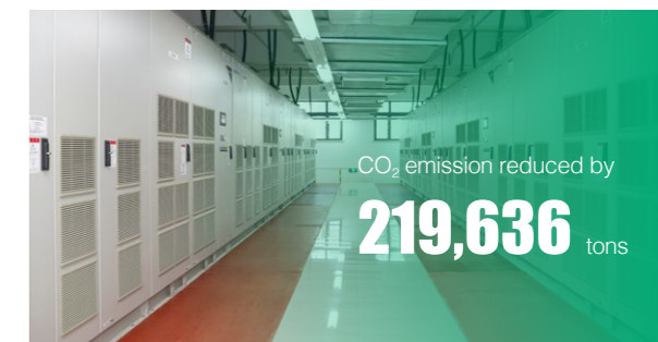
Hengli Petrochemical Refining frequency converters
