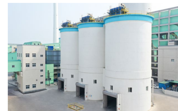
Hengli Petrochemical Refining fly ash recycling system
